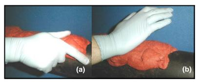
Figure 3-30: Applying the DMP-3 Material
